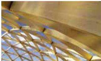
**MAINTENANCE AND CORROSION** \_Timber glue laminated beams are proven resistant in salty environments. Minimal maintenance is guaranteed as wood is a non-corrosive material.
